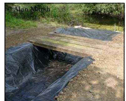
The emergency overflow after cutting a new channel and re-lining
