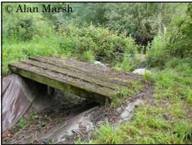
The emergency overflow before restoration: the bank had eroded under the liner
